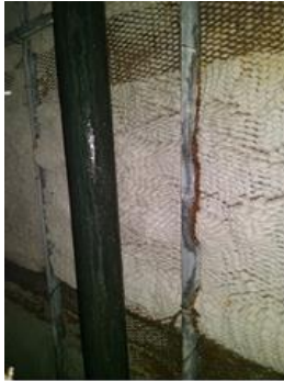
Missing insulation on cold water riser
