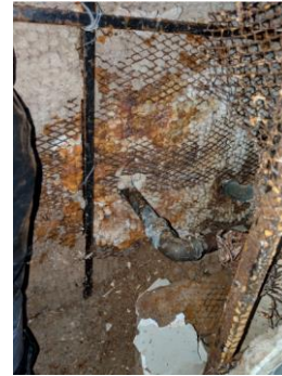
Missing insulation on cold water supply t
