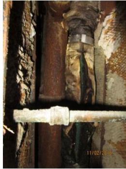
Damaged insulation on cold water riser
